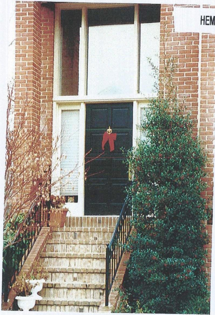
FRONT ENTRY DOOR, Townhouses (8-panel wood door painted black, dark green, trim color, or semi-transparent stain.)
