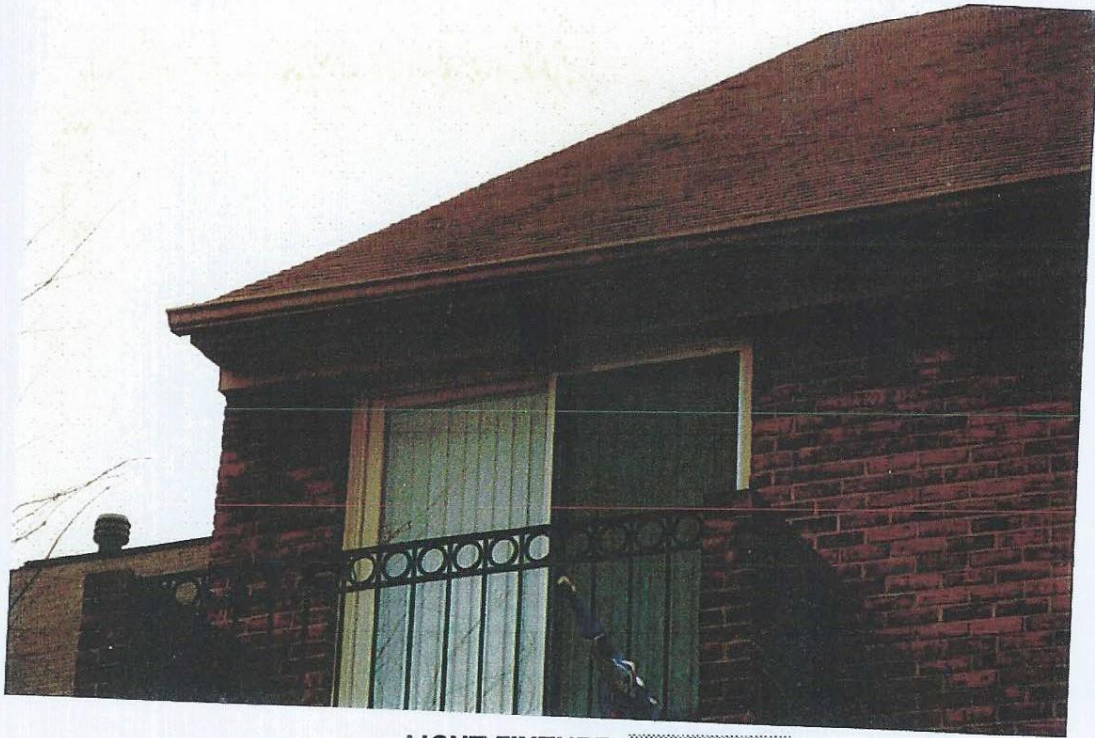
LIGHT FIXTURE, Townhouses
