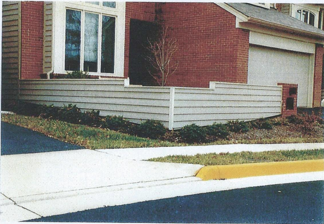
COURTYARD FENCE, Patio homes only (Same color, details, and materials as house siding. See specification sheet on reverse.)
